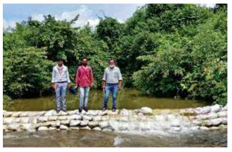
Boribandh is a low cost water harvesting structures used for the harvesting of rain water. 3,960 boribandhs have been constructed.
